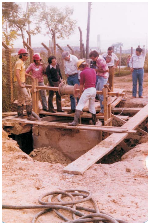
Figure 11 - Trial shaft for the River Tietê tunnel.
